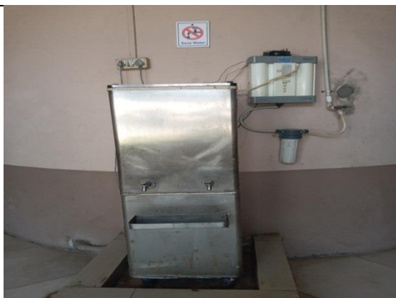
Water cooler with RO system
