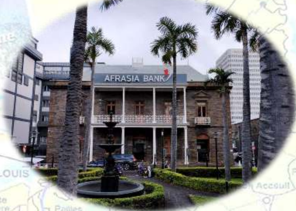
Afrasia Bank Building, Port Louis
