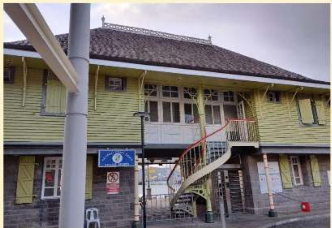
National Coast Guard Head Office Building, Port Louis
