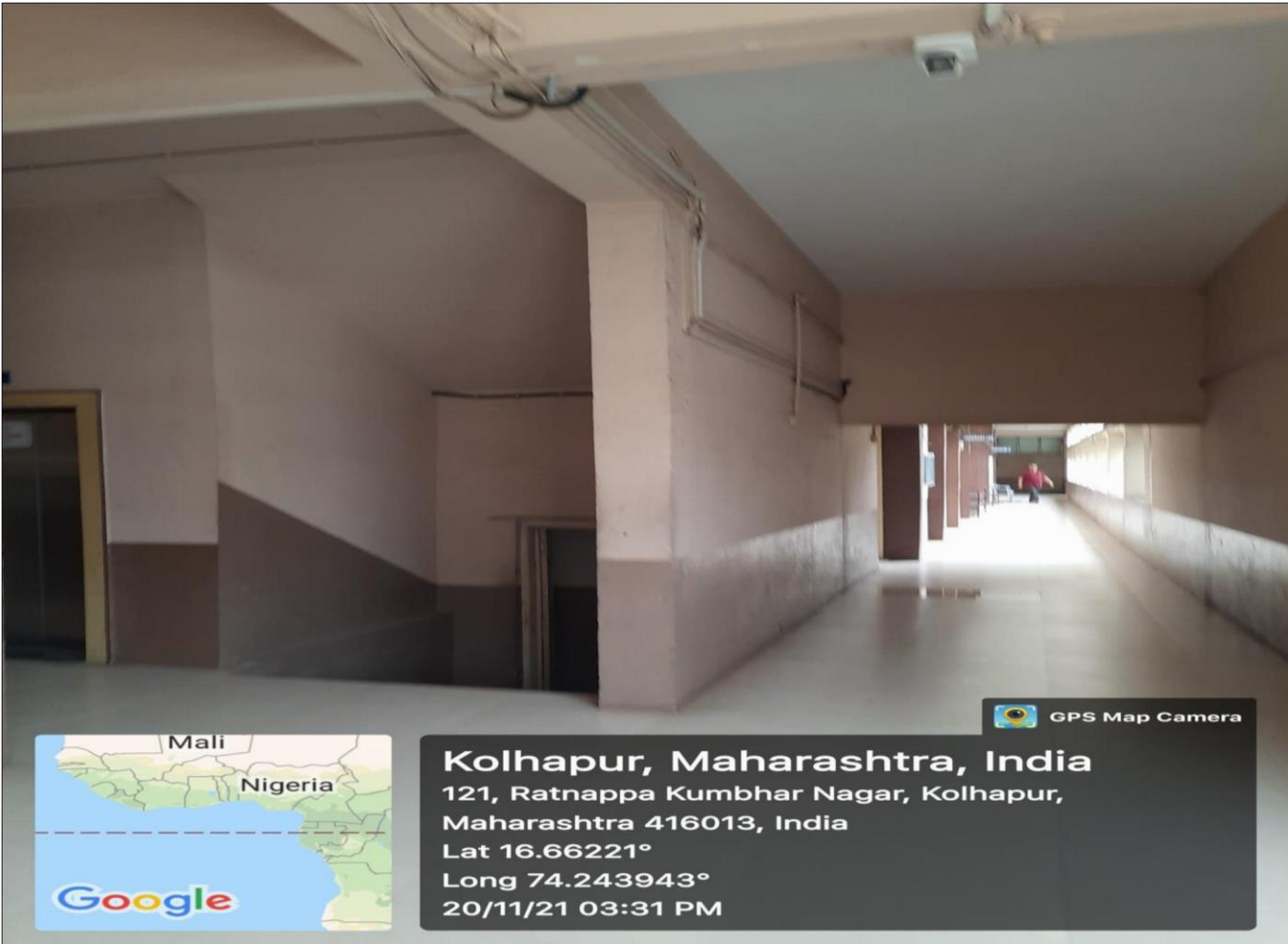
CCTV Ground Floor
